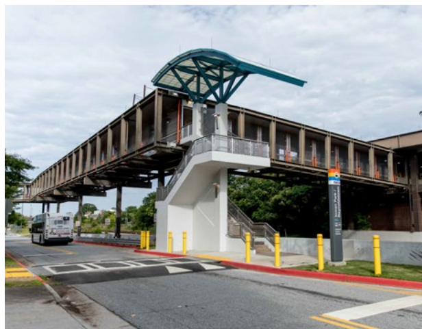
Reynoldstown Bridge: Before and After
